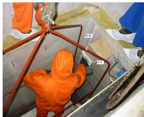
Fig. 4 - Former spent fuel pool
