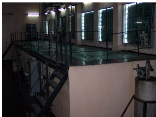
Fig. 3 - Former spent fuel disposal building
