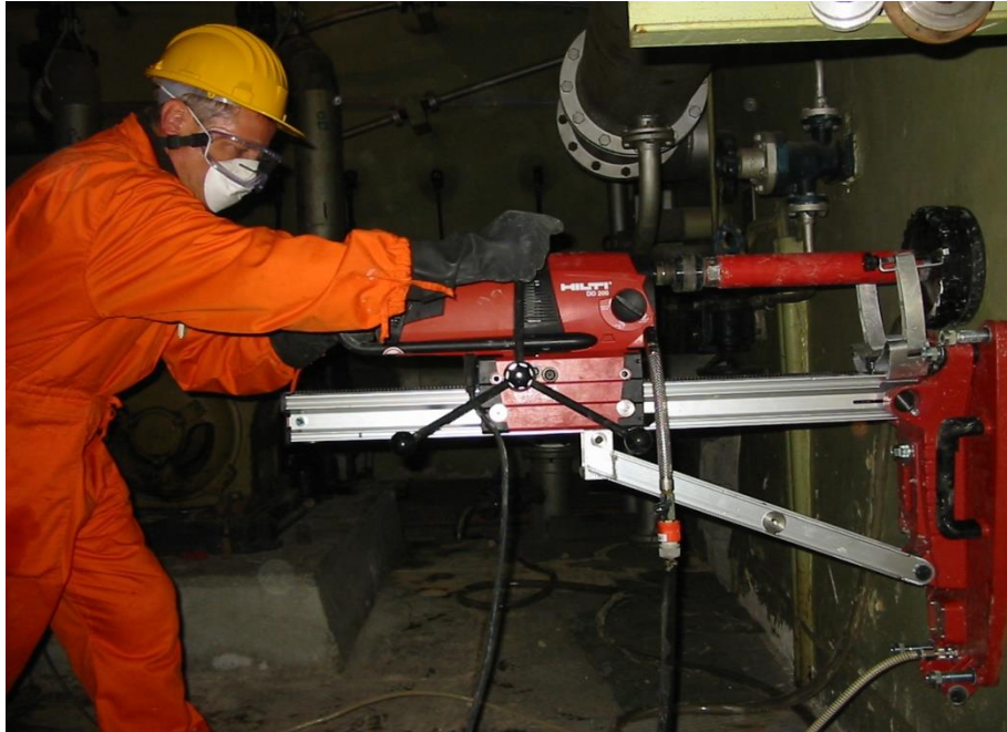
Fig. 5 Diamond drill equipment for concrete core extraction - DD200
